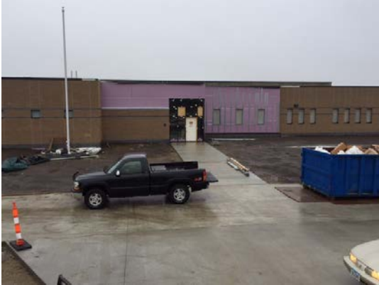
Patrol building construction
